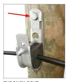
**THROUGH BOLT:** In this case, the suspension clamps are directly secured to the pole using a through bolt at all intermediate poles \*with angles less than 20° and perpendicular to the cable route.
