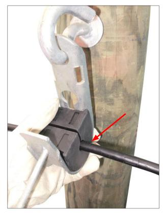
**STEP 5:** Place the cable inside the neoprene sleeve back into the clamp body.
