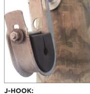
In this case, the suspension clamps are directly secured to the pole using a J-hook at all intermediate poles \*with angles less than 20° and perpendicular to the cable route
